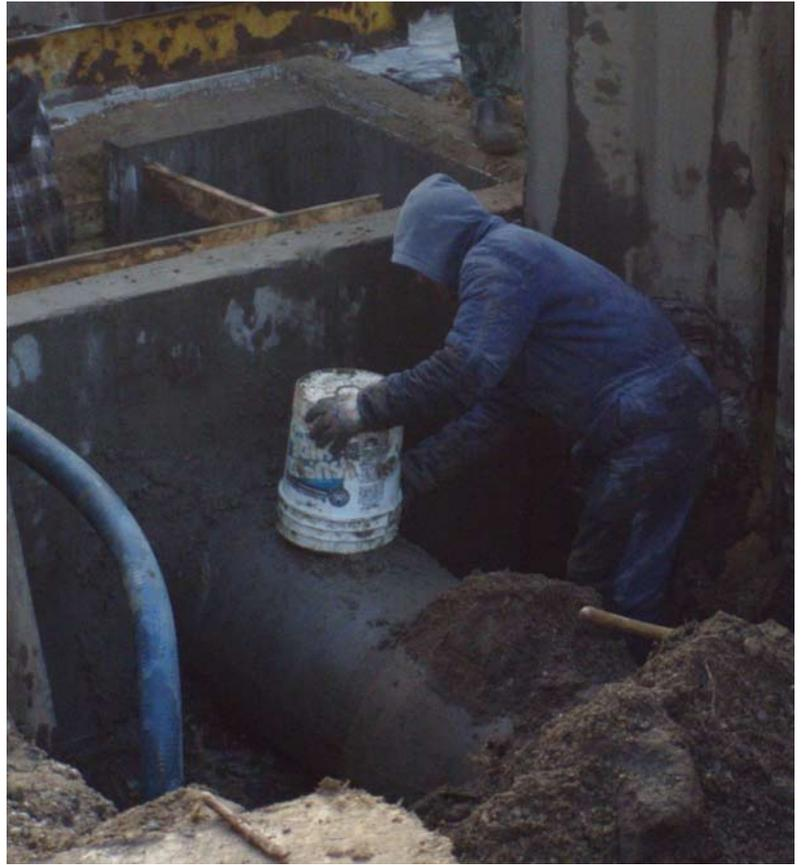
Sealing the connection from the outside of the outflow box.
