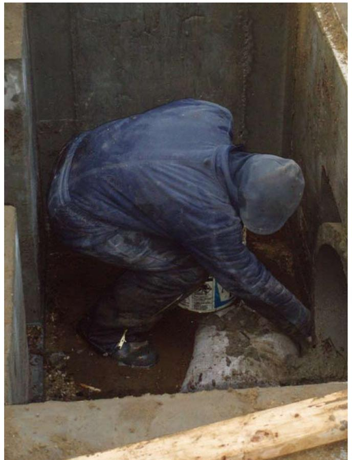
Sealing the connection from the inside of the outflow box.
