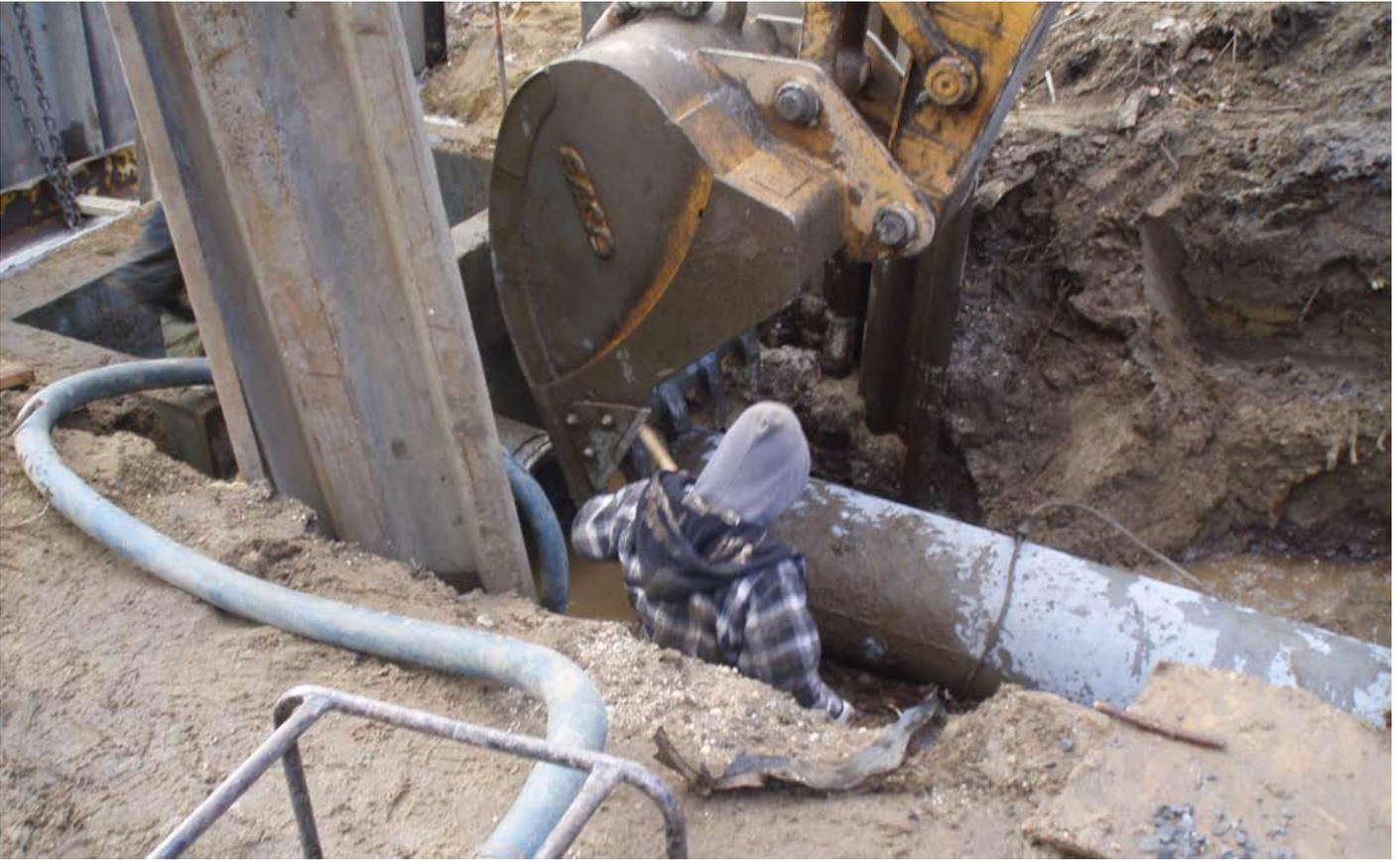
Connecting the new outflow box to the pipe.
