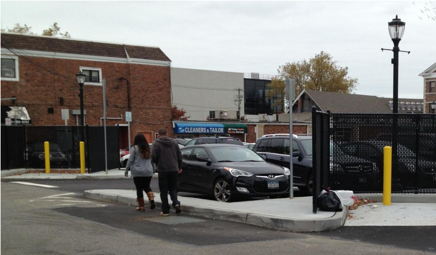
Figure 27 Poor Pedestrian Access at Newly Renovated Town Lot
