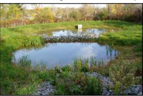
Stormwater retention ponds provide effective water quality control by using forebays for sediment settling, and have controlled-discharge outlets for flood control.
