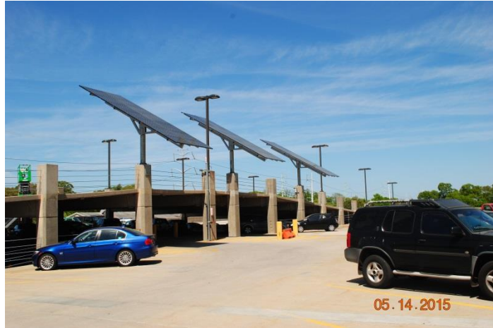
Solar panels at LIRR South Parking Garage that supply energy to electric car charging stations located within it Huntington
